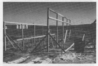
Tables 30" high  $\times$  36" wide running the full length of the building are made along the side walls. And one table 30" high  $\times$  72" wide is made down the center. The aisles between the tables are  $3\frac{1}{2}$  wide. (If your seedling greenhouse is smaller, you may skip the center table.)
