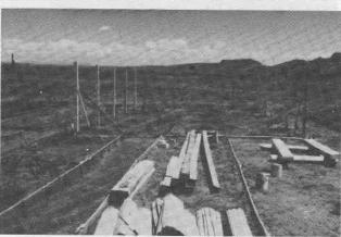
The posts for the sides of the building are 8' long and are set in the ground 18" below the level of the floor.
