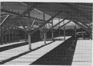
To complete the tables, nail  $1\times4$  boards 36'' long on top of the  $2\times4s$  on the side tables, and  $1\times4$  boards 72'' long to complete the center table.
