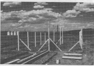
The first step in construction is to clear and level the area. Then set stakes for the  $4\times4$  posts. The posts are 10' apart each direction.
