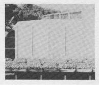
Special plastic materials are available to cover greenhouses. The clear plastic is pulled over the top of the building as one sheet. Lath is placed on top of the plastic along the rafters and nailed to the rafters. This secures the plastic.
