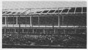
...and the bottom-end is nailed to a  $1'' \times 8''$  board which is nailed along the outside edge of the building near the floor level.
