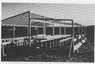
The top-edge of properly placed  $2\times4$  table legs is level throughout and in a straight row. The next step is to nail  $2\times4$ s on edge on top of each row of table legs.
