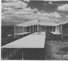
To strengthen, stabilize, and secure the greenhouse, pieces of lumber such as  $1\times4s$  48" to 60" long are used for cross braces. The braces are nailed to the posts, rafters, and stringers.
