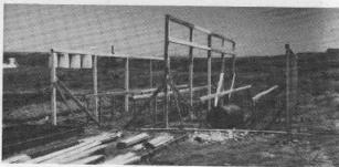
The center table is made just like the side tables. There are two rows of legs 30" away from the center  $4\times4$  posts, one row on each side of the posts. A third row of legs is in line with one edge of the  $4\times4$  posts. The legs in this row are 24" apart.
